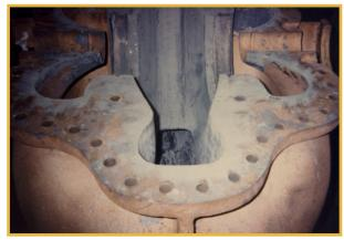
SC3910 is a two-component 100% solids trowel-grade epoxy novolac caulk for use as a chine repair or lap weld feathering product for steel tanks. It is often used in conjunction with chemical-resistant topcoats such as SC3300 or SC5400. It offers excellent chemical resistance to a wide range of petrochemical products, fuels, organic/inorganic acids and alkalis. A long re-coat window allows it to be top-coated up to 14 days, depending on temperatures.
